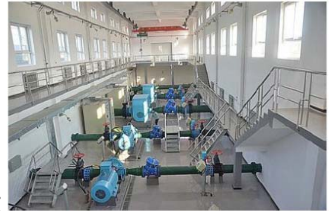
Figure 5-71 Backwash Pump House
